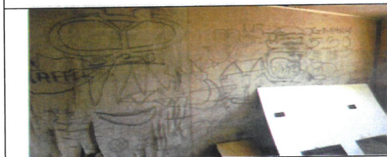
Fig 5.0 View showing all rotten wall cladding to be remove and replace with new. Room 1. Duplex 1
