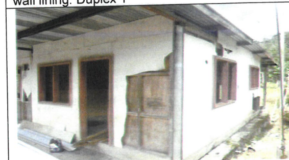
Fig 17.0 View of SOQ 1, Duplex 1 & 2 showing all external cladding to be remove and replace with new.
