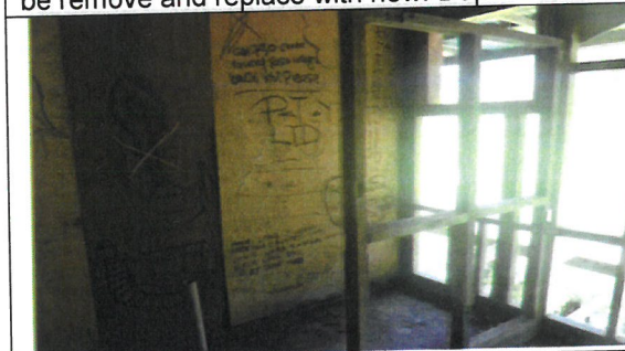
Fig 15.0 View showing missing frames without wall lining. Duplex 1
