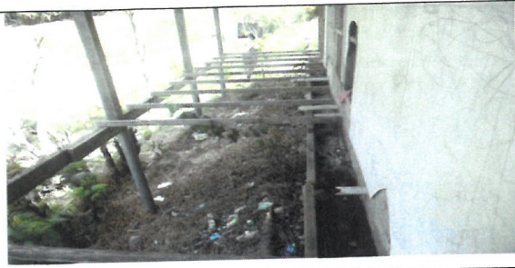
Fig 9.0 View showing back view of poor verandah rails, with no floor joist and flooring. SOQ 1, Duplex 1 & 2. Verandah.
