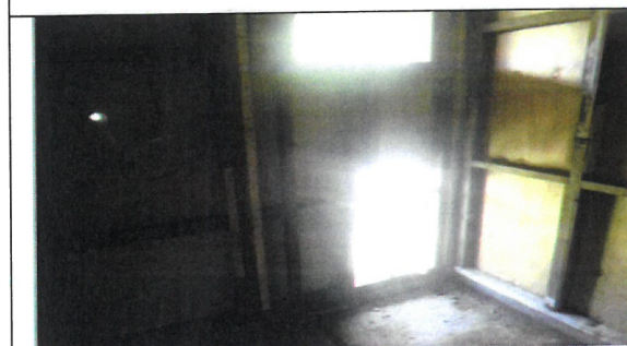
Fig 7.0 View showing rotten studs, rotten noggin, and wall partition to be remove and replace with new. Toilet and bathroom. Duplex 1
