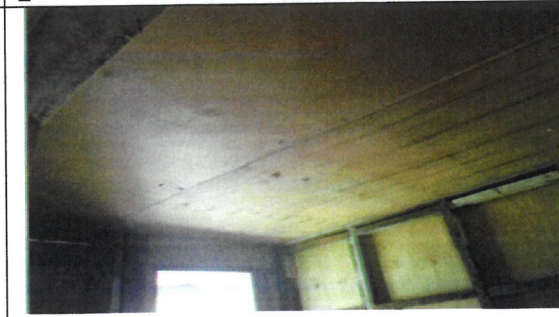
Fig 8.0 View showing rotten ceiling lining to be remove and replace with new. Living room. Duplex 2.
