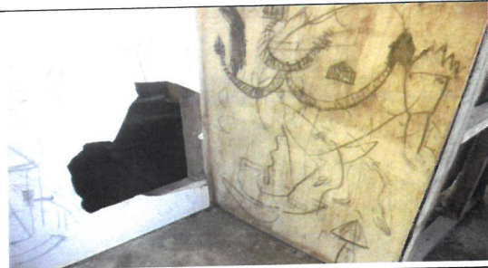
Fig 10.0 View showing broken wall cladding to be remove and replace with new panel rib color bond. External view.
