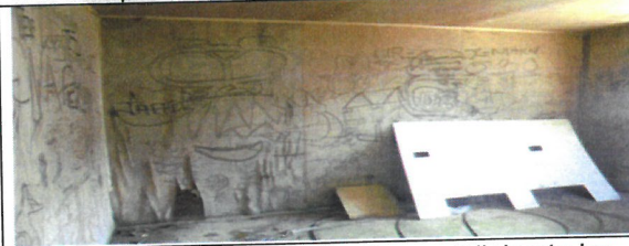
Fig 14.0 View showing all rotten wall lining to be remove and replace with new. Duplex 2
