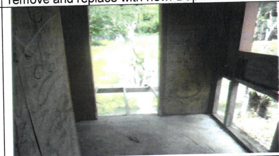
Fig 16.0 View showing no proper door frames and Window frame. Duplex 2
