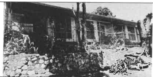
Fig 2.0 View showing poor fencing at the retaining wall. To be remove and reconstructed with new spike fencing.
