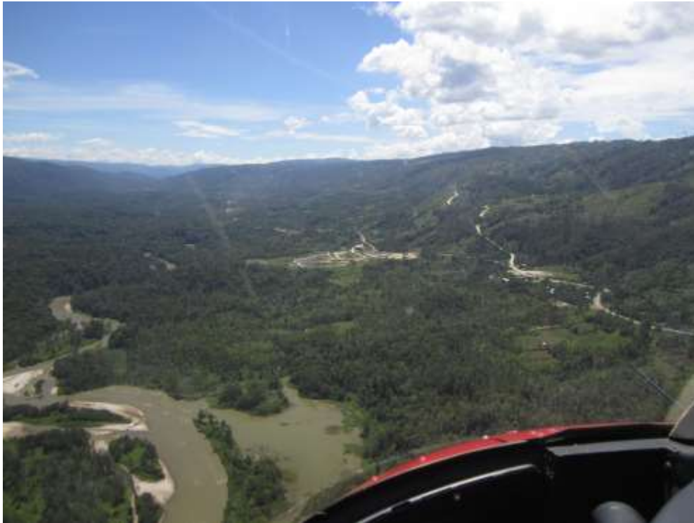
▲ Photo 1 – Aerial view of road (on right) leading from Hides Gas Generation Station to Hides Gas Conditioning Plant (~13km). Togari River (looking downstream) on left.
