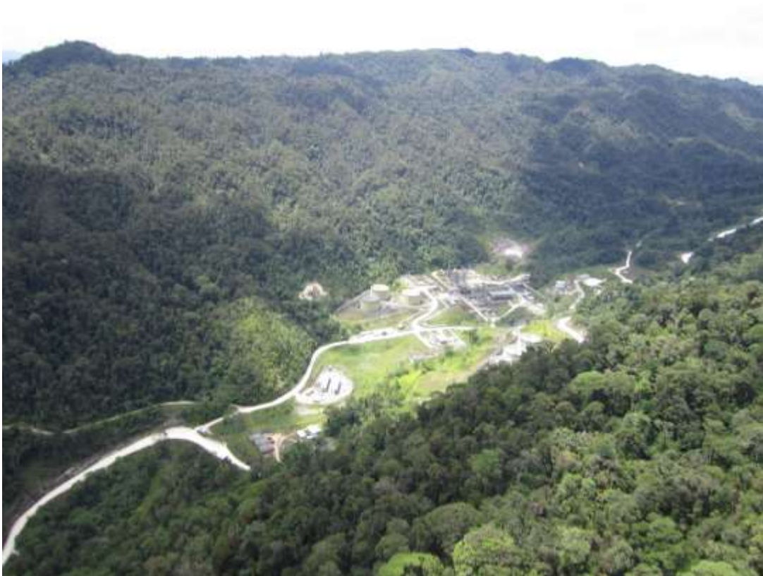
Figure 4: Existing Kutubu Central Gas Processing Plant
