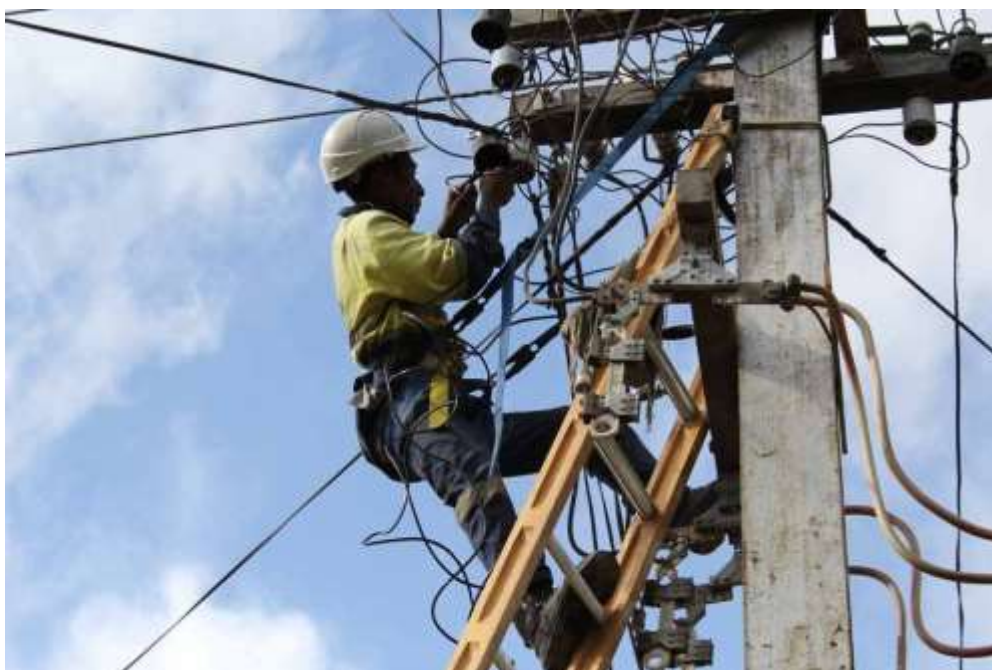
Figure 1: PPL Linesman working on Existing MV Distribution Network
