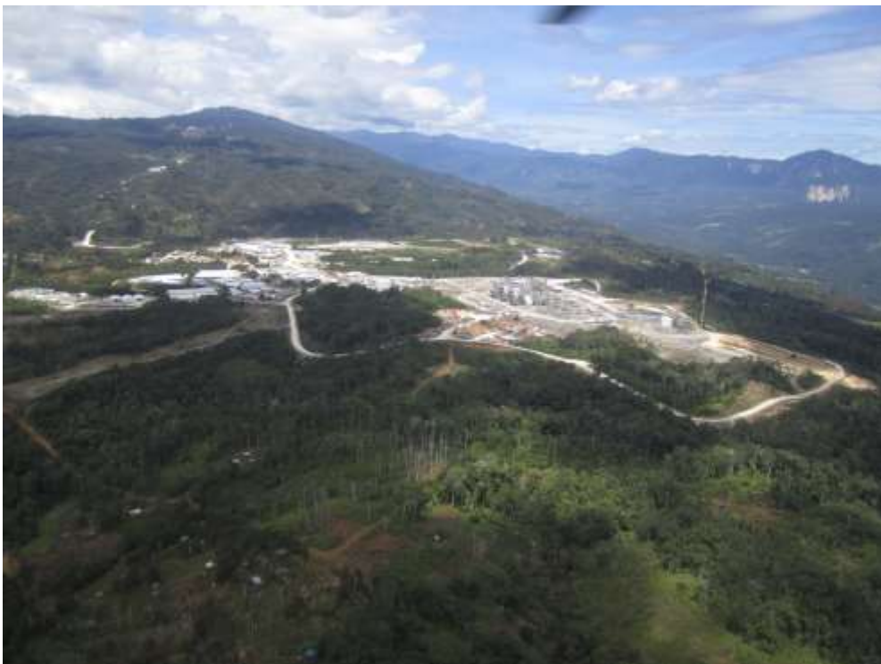
▲ Photo 2 – Hides Gas Conditioning Plant (Hides Gas Generation Plant located in the valley ~13km straight ahead over the ridgeline).
