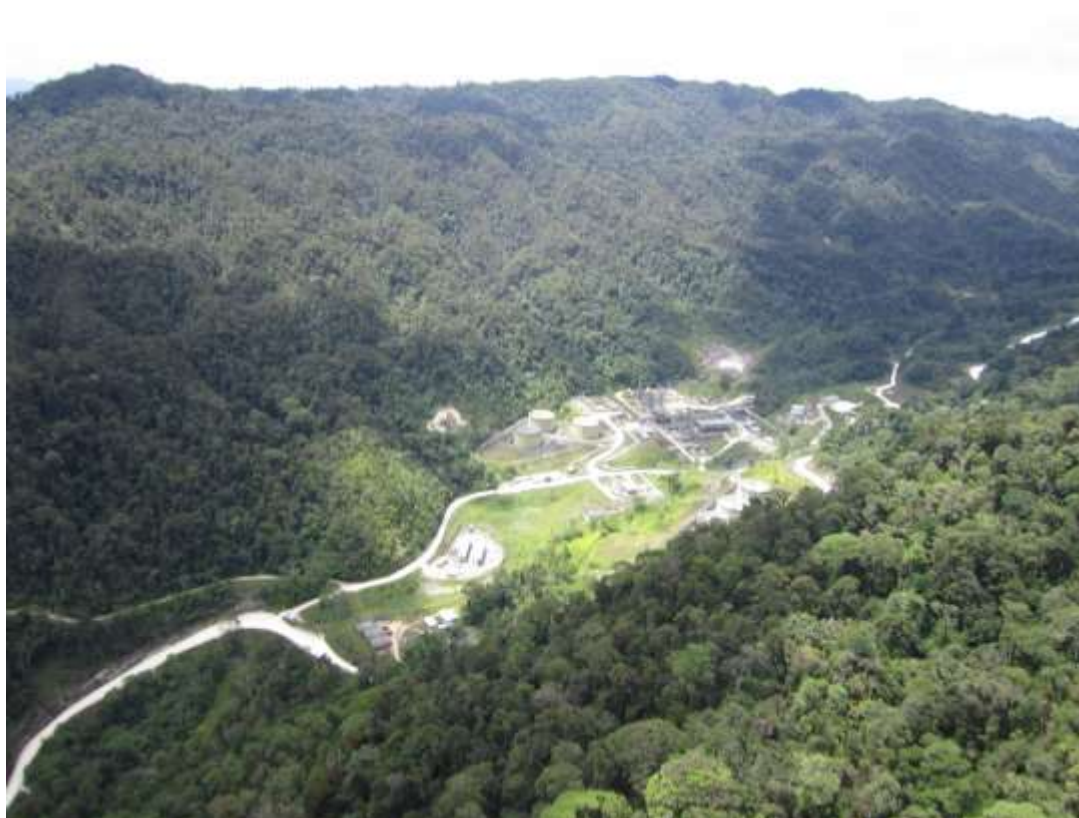
Figure 4: Existing Kutubu Central Gas Processing Plant
