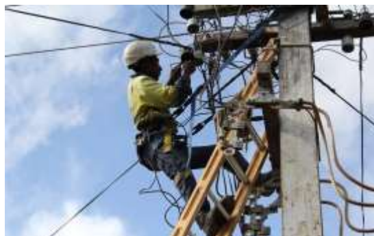
PPL Linesman at work on MV distribution system
