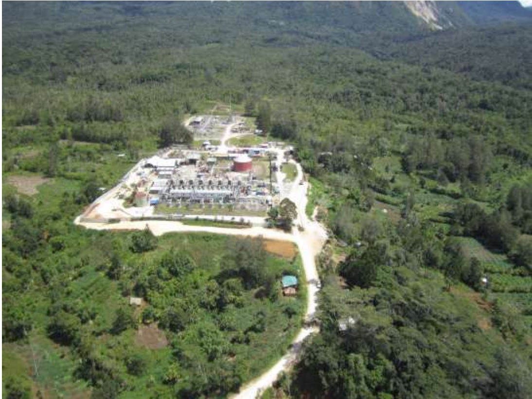
Figure 3: Existing Hides Gas Generation Plant
